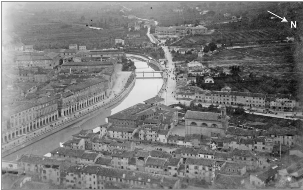
Figure 1. Aerial photo of the Rione Porto (Senigallia). Notice the collapse of roofs and the widespread damage to buildings. The church of Santa Maria del Ponte al Porto and its damaged bell tower is seen in the foreground. The Portici Ercolani are shown on the left side of the image (on the right bank of the Misa River). This rare photo was taken by the air squadrons of the 20th Stormo of the Aeronautica Militare Italiana immediately after the earthquake.
