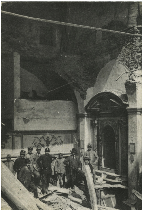
Figure 2. The very ancient church of San Giacomo of Citerna heavily damaged by the earthquake of April 26, 1917.
